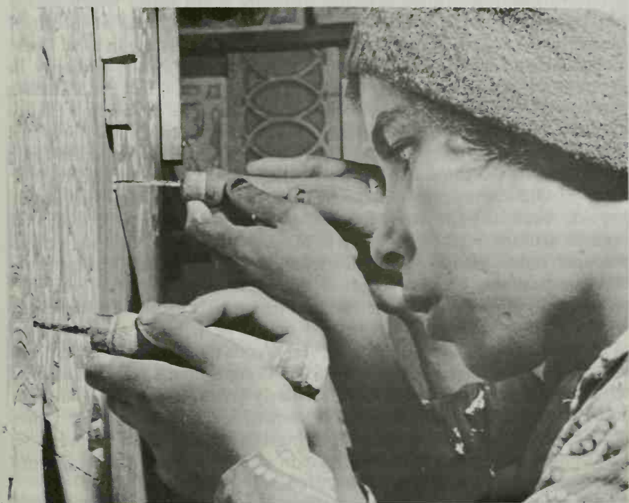
The most delicate operation: piercing the plaster.
