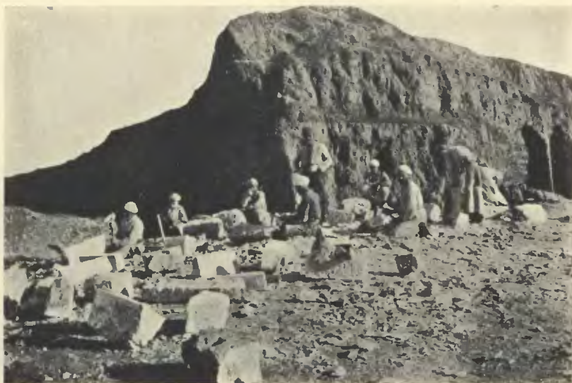
Excavation of stones from the foundations of Sennacherib's wall between Kuyunjik and Nabi Yunis.
