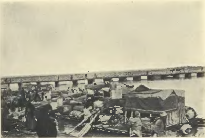
The new bridge over the Tigris at Mōsul.
