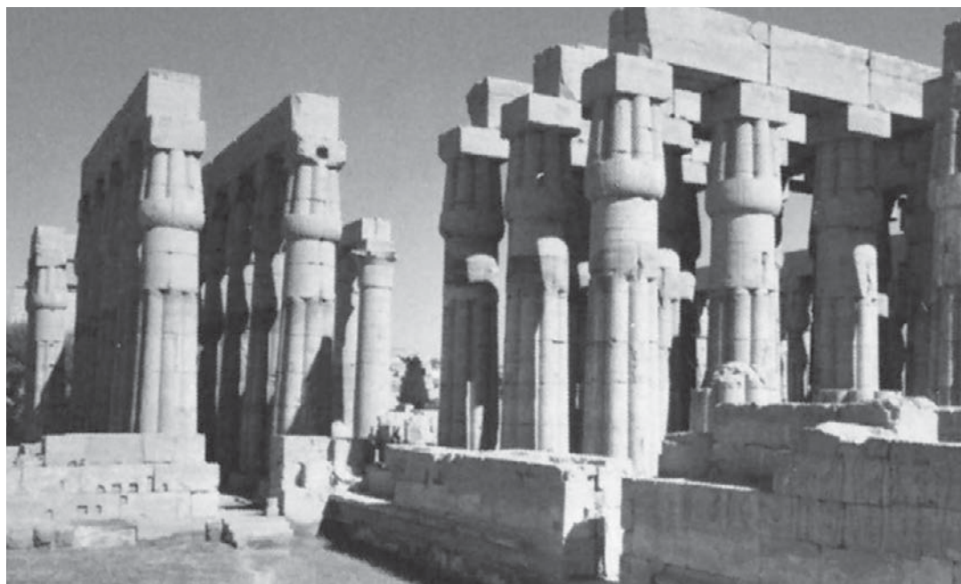
Papyrus-cluster columns of the peristyle forecourt of the Temple of Luxor (seen from the southwest) in Thebes, Egypt. The 18th- to 19th-dynasty structure was built by Amenhotep III about 1390 BC and is sometimes called the Great Temple of Amon, though that name is normally reserved for the larger temple complex at nearby Karnak. Hirmer Fotoarchiv, München
