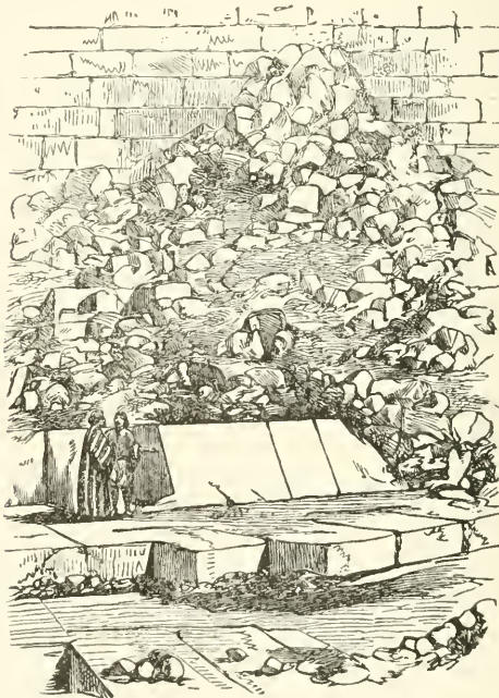
Fig. 54.—OUTER CASING STONES OF THE GREAT PYRAMID.—See Page 101.
