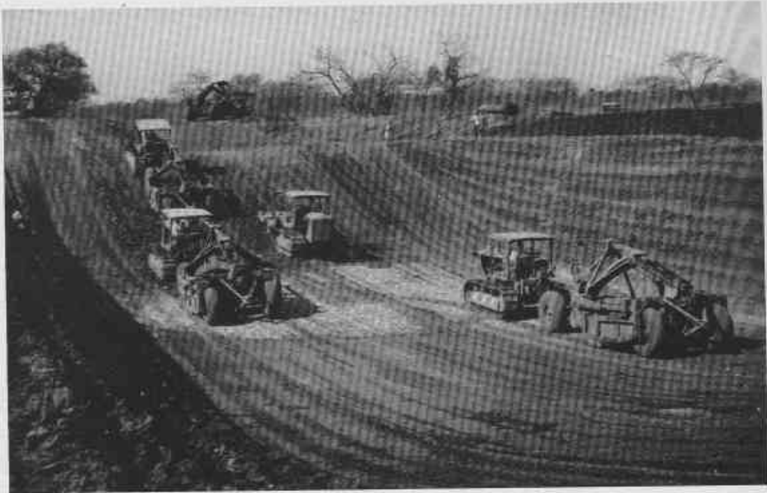
PLATE XXX. HAFIR -EXCAVATING TEAM AT WORK
