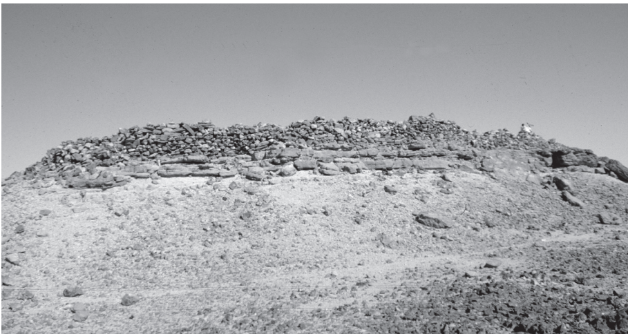
Figure 3: External wall of the late Roman hill-top fortress in the north-eastern part of Wadi el-Hudi, photographed from the west. (WH92/77).
