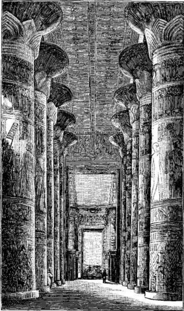
GREAT HALL OF COLUMNS AT KARNAK (RESTORED.)
