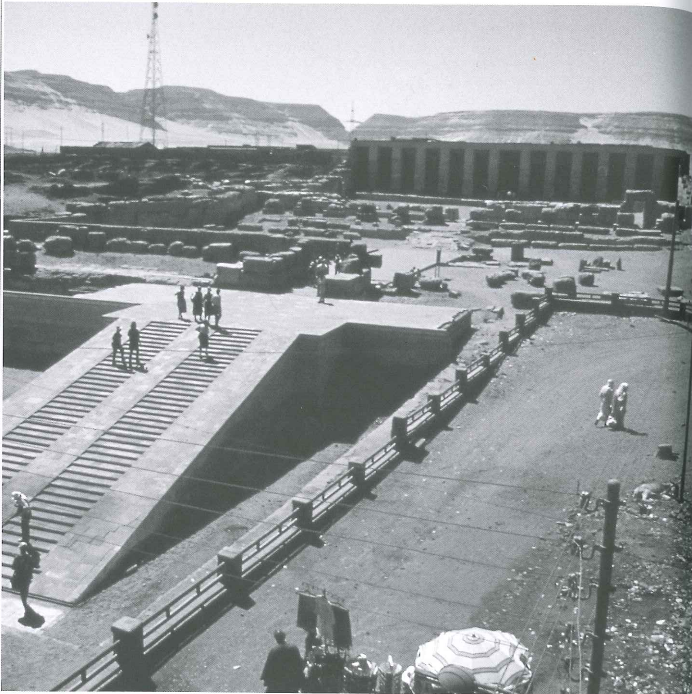
13 View of the pillared façade of the Seti temple.
