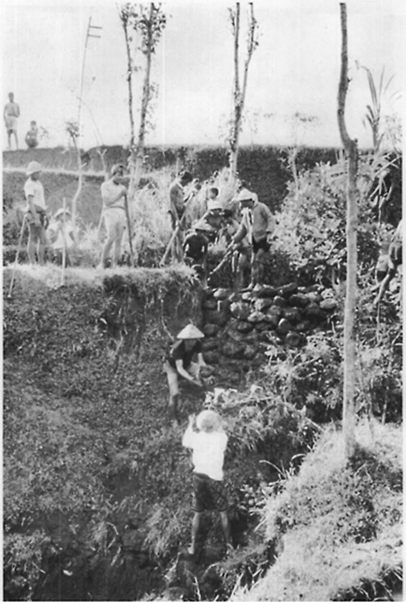
10. Repairs on minor damage to an irrigation channel in Subak Langkih
