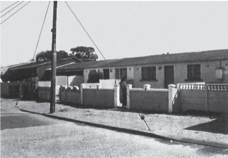
FIGURES 3.1 AND 3.2: Typical street and council houses in Guguletu township Source: Japha, Derek and Marie Huchzermeyer, 'The history of the development of townships in Cape Town, 1920–1992', The Integration and Urbanisation of Existing Townships in South Africa Working Paper no. 2 (Newcastle and Cape Town, 1995)
