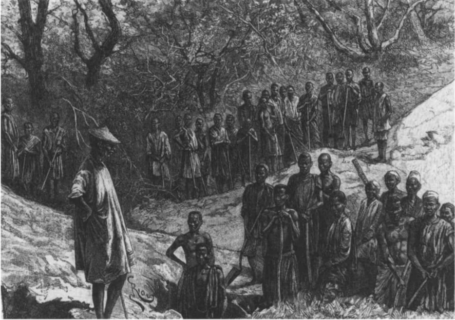
Fig. 9 Forced labour levy gets ready to work on railroad construction.
