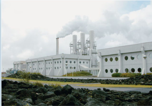
FIGURE 11.1.2 Svartsengi geothermal power plant. On the Reykjavík Peninsula, southwest of Iceland’s capital, the Svartsengi power plant produces electricity and provides hot water for homes and businesses. The plant’s name means “Black Meadow,” referring to the extensive lava beds throughout this region of Iceland. [Bobbé Christopherson.]
