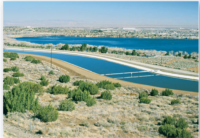
(b) California Aqueduct
