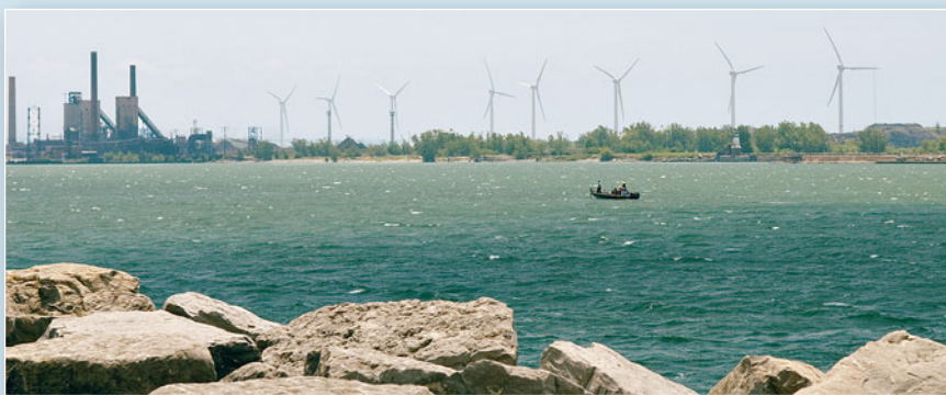
FIGURE 6.1.2 Wind turbines at a former industrial site.
