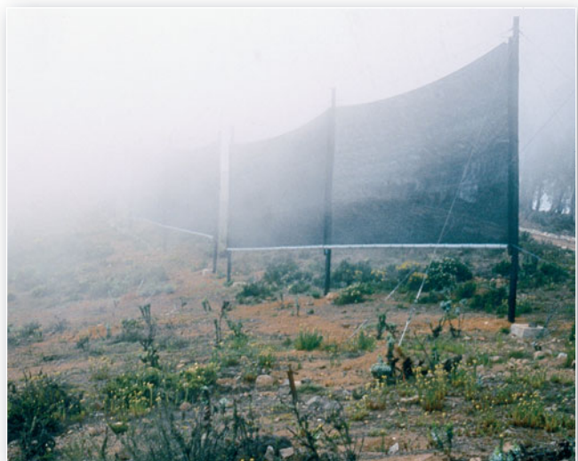
FIGURE 7.24 Fog harvesting. In the mountains inland from Chungungo, Chile, polypropylene mesh stretched between two posts captures advection fog for local drinking-water supplies. [Robert S. Schemenauer.]
