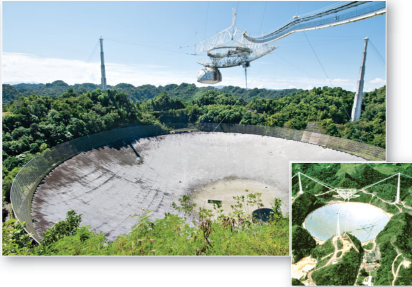
FIGURE 13.19 Deep-space research using cockpit karst topography. Cockpit karst topography near Arecibo, Puerto Rico, is the setting for Earth’s largest radio telescope. The discoloration of the dish does not affect telescope reception. The suspended movable receivers where the signals focus are 168 m (550 ft) above the dish. [Bobbé Christopherson; inset Cornell University.]
