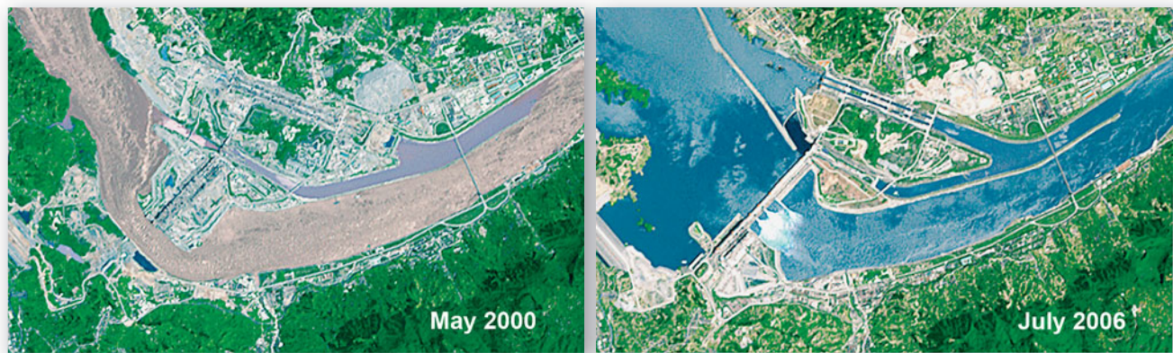
FIGURE 9.12 Major dam in China.
