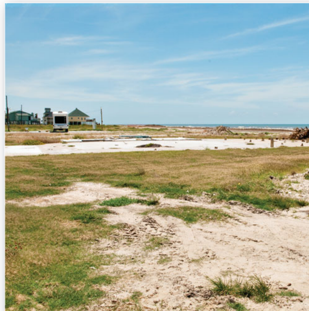
(c) Empty foundation pads, houses gone
