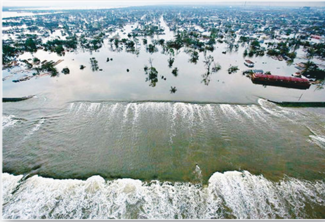
FIGURE 14.24 Levee break and devastation in New Orleans.
