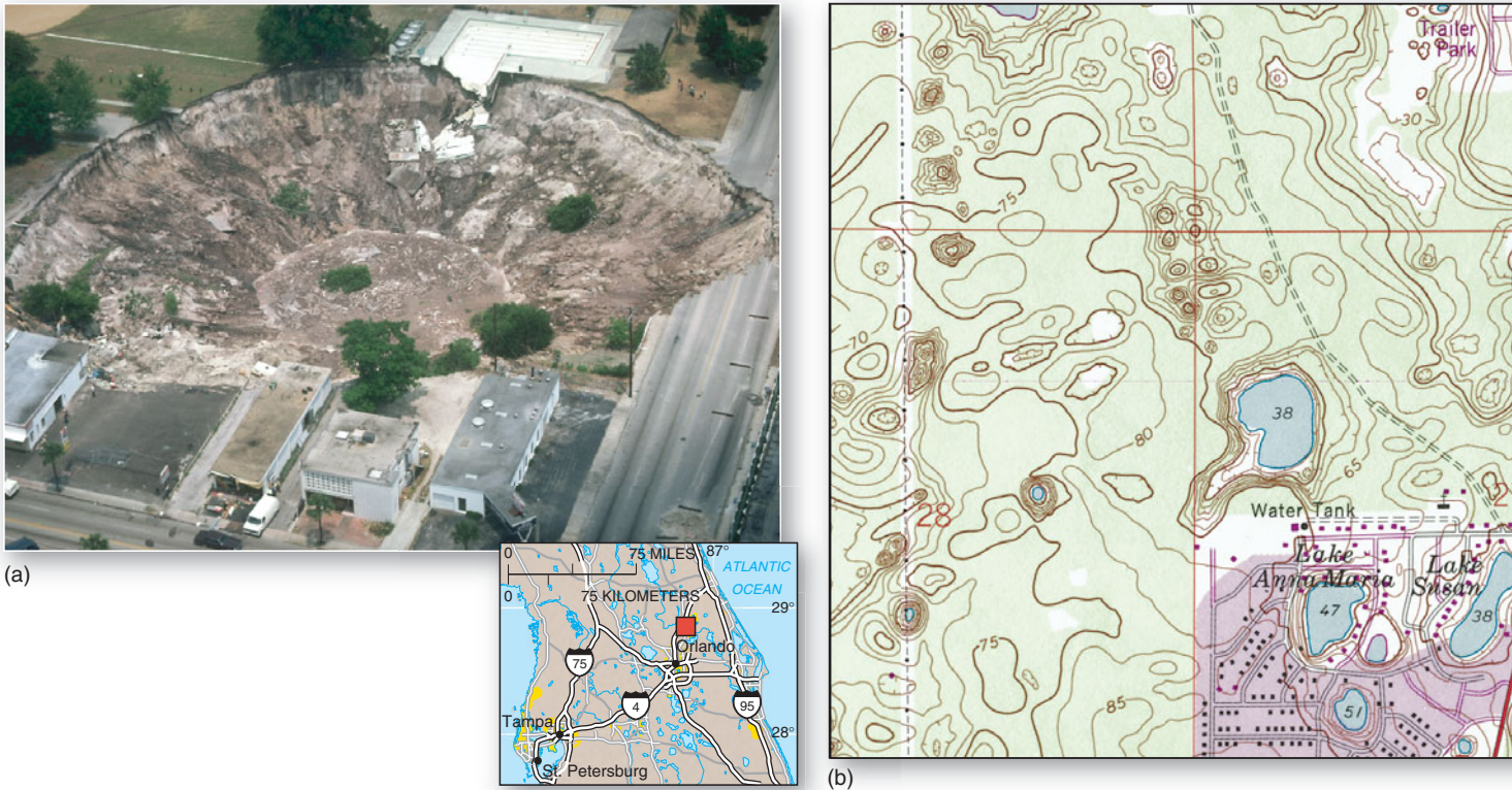
FIGURE 13.17 The Winter Park sinkholes.
