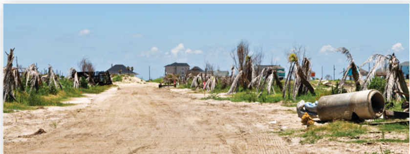
FIGURE GN 8.2 Hurricane Ike swept away all homes and the pavement in this neighborhood. Many kilometers of coastline were destroyed on Bolivar Peninsula, Texas. [Bobbé Christopherson.]
