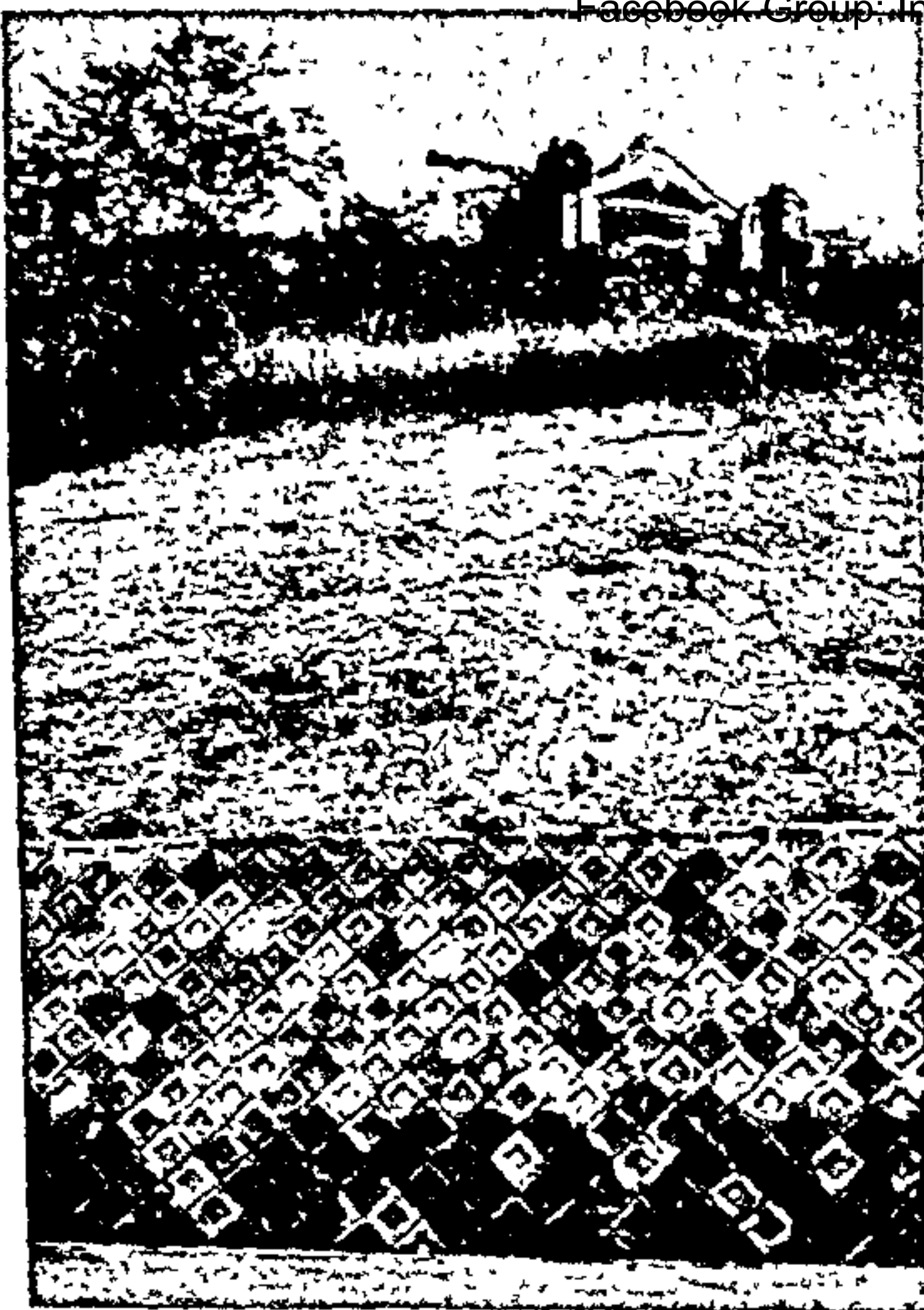
4.D An effective way of preventing landslide by building a concrete wall—Taiwan Goh Cheng Leong
