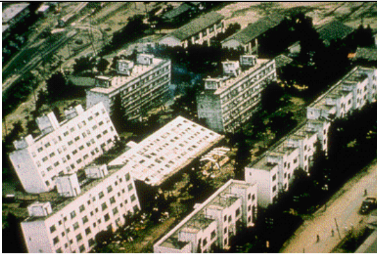
{PRIVATE} Figure 10m-7: Earthquake of June 16, 1964 in Niigata, Japan had a magnitude of 7.4. Liquefaction of some soils in the area caused large apartment buildings to tip over on their sides. ( Source: Image provided by the National Geophysical Data Center, NOAA ).
