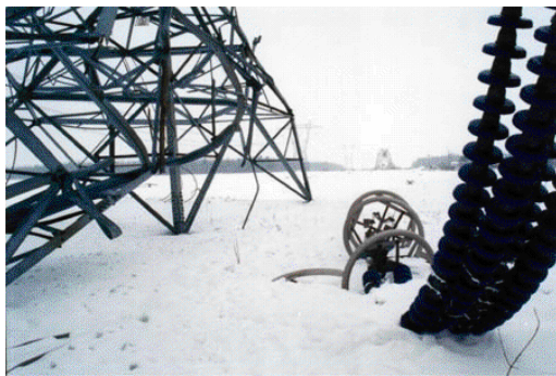
Figure 7s-6: The weight of ice collapsed many power-transmission towers leaving some areas without electricity for almost two weeks. (Source: Human Resources Development Canada - Ice Storm '98 Emergency: A Study in Response ).
