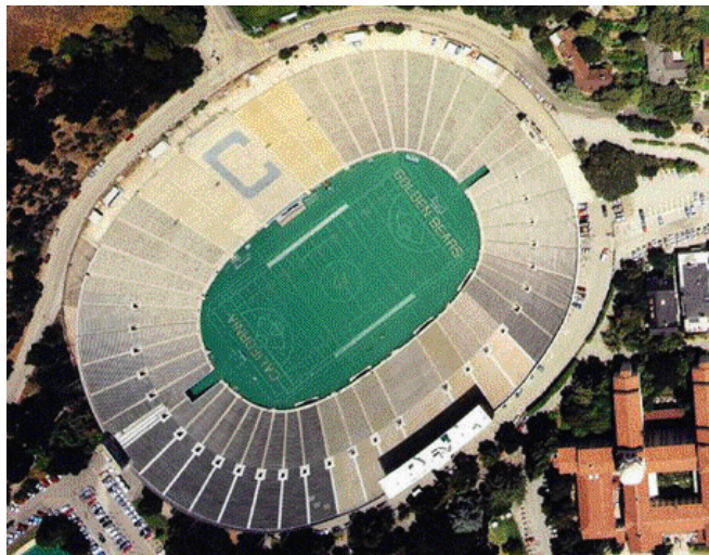
{PRIVATE} Figure 2e -9: Football stadium at the University of California at Berkeley. Football stadiums have an obvious shape that can be easily recognized even from vertical aerial photographs. (Source: University of California at Berkeley - Earth Sciences and Map Library ).
