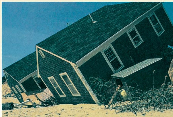
▲ Coastal erosion Wave action has undermined the bluff beneath these two buildings, depositing them on the beach below.
