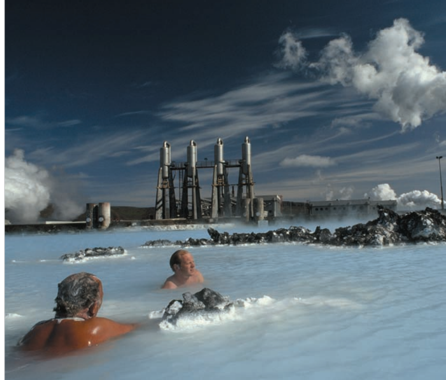
Geothermal power plant FIGURE 9.11
