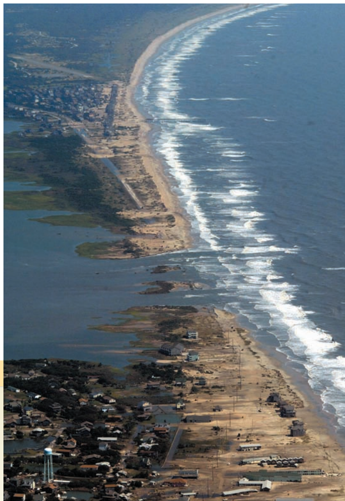
▲ New inlet Storm waves from Hurricane Isabel breached the North Carolina barrier beach to create a new inlet, as shown in this aerial photo from September 2003. Notice also the widespread destruction of the shoreline in the foreground, with streaks of sand carried far inland by wind and wave action. As sea level rises, ocean waves will attack barrier beaches with increasing frequency and severity.
