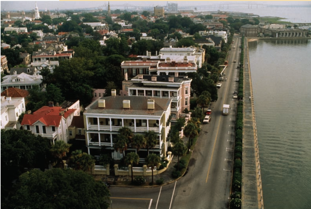
▲ Charleston, South Carolina These old homes on the Charleston waterfront display a local architecture well adapted to the climate of the region. The upper porches were used for outdoor living and sleeping in the hot and humid summer weather. (Charleston is located on Figure 7.23.)
