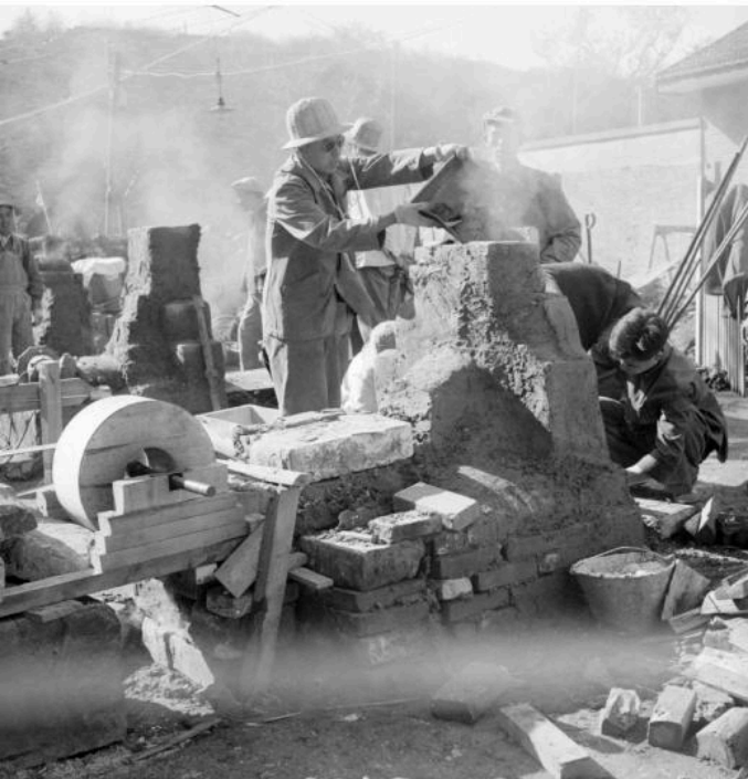
▲ Constructing a rudimentary smelting steel furnace, 1958
