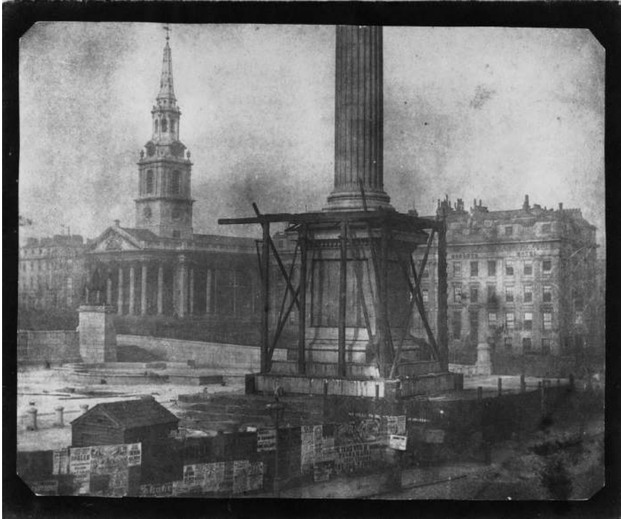
Figure 10.9 William Henry Fox Talbot, Nelson's Column under Construction in Trafalgar Square, London , April 1844. Digital image courtesy of Getty's Open Content Program.
