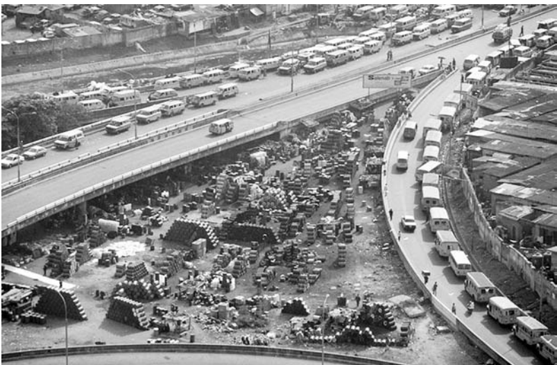
FIGURE 14. Lagos 2000. The traffic jam on the bridge and repair shops beneath. Source: Edgar Cleijne; used by permission.
