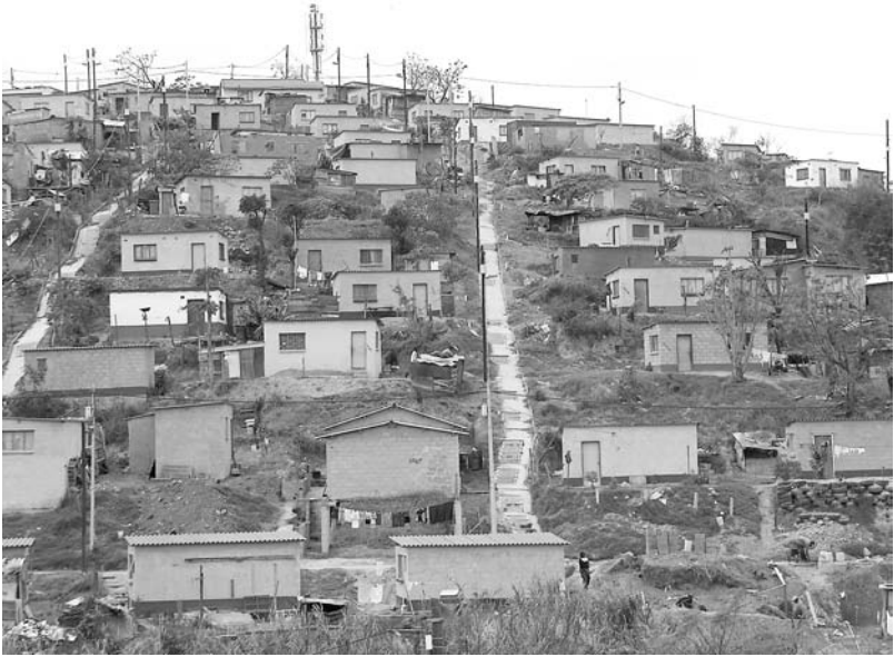
FIGURE 18. Cato Manor, South Africa. Post- apartheid 'RDP' state-subsidised housing. Source: Stéphane Vermeulin; used by permission.
