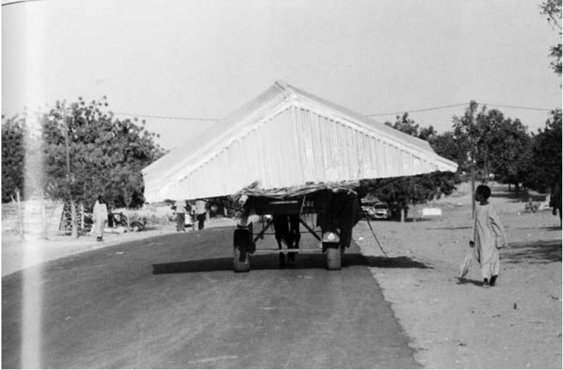
FIGURE 15. Roof delivery: how Touba is being constructed. Source: Dr. Cheikh Guèye; used by permission.
