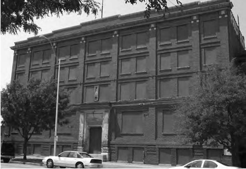
Figure 5. The Paseo Street YMCA in Kansas City's black district, where the Negro National League was founded in 1929. Today it is a merely an eyesore, a blighted brick building located just two blocks from the gleaming Negro League Museum.
