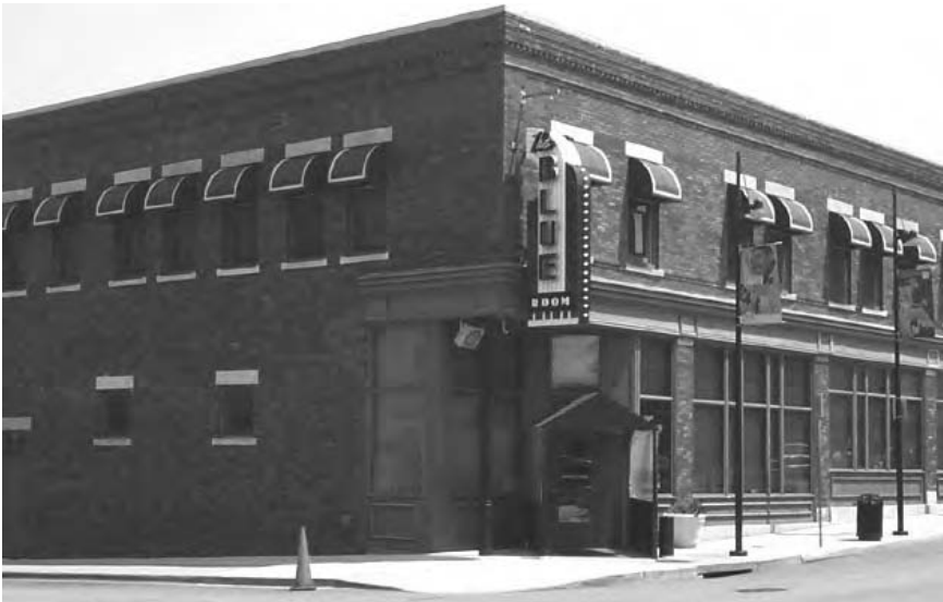
Figure 6. The Blue Room restaurant stands where The Streets Hotel once thrived as a nexus of black community life in 18th-and-Vine section of Kansas City.
