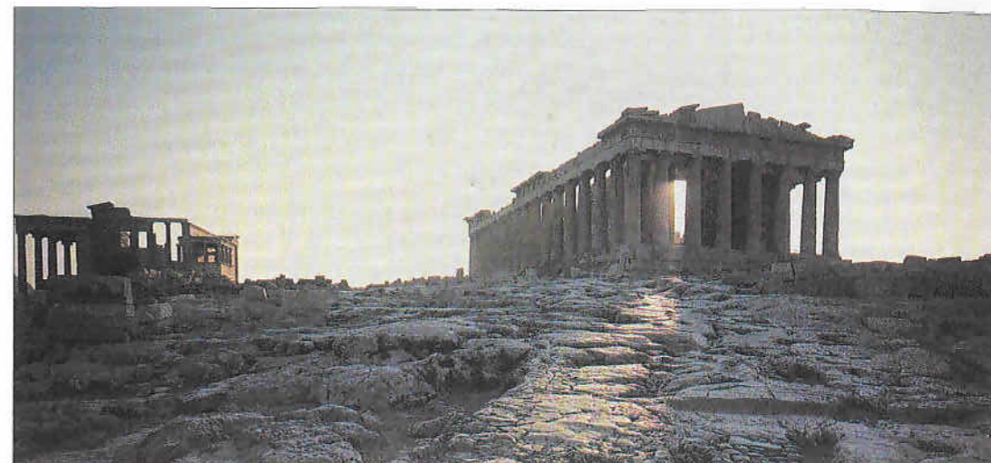
The Parthenon and, to the left, the Erechtheion with its caryatid porch. Just under 70 by 30-metres in plan, the Parthenon was designed by the architect Iktinos, who worked with Athens' master-builder Kallikrates. This beautiful building stood intact with all its sculptures until 1687 when a Turkish powder-magazine within its walls was ignited by a shell fired by a Venetian artillery battery besieging the city.
