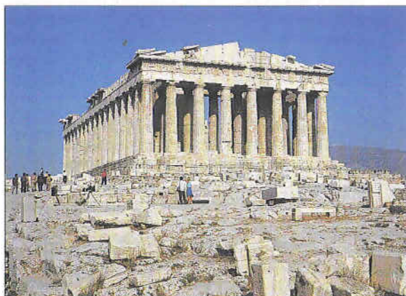
Perhaps the single greatest architectural symbol of the Athenian Golden Age under Perikles is the Parthenon which surmounts the Akropolis. In its design and execution the Parthenon is a classic Doric temple, veering away from tradition only in its possession of an exquisitely-carved frieze which ran along the top of the wall within the outer colonnade.
