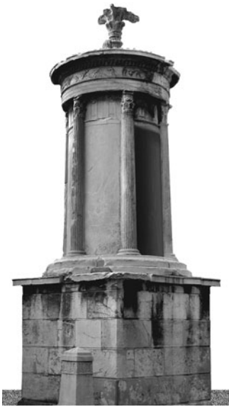
Fig. 8a The choregic monument of Lysikrates with open front in the intercolumniation facing the road.
