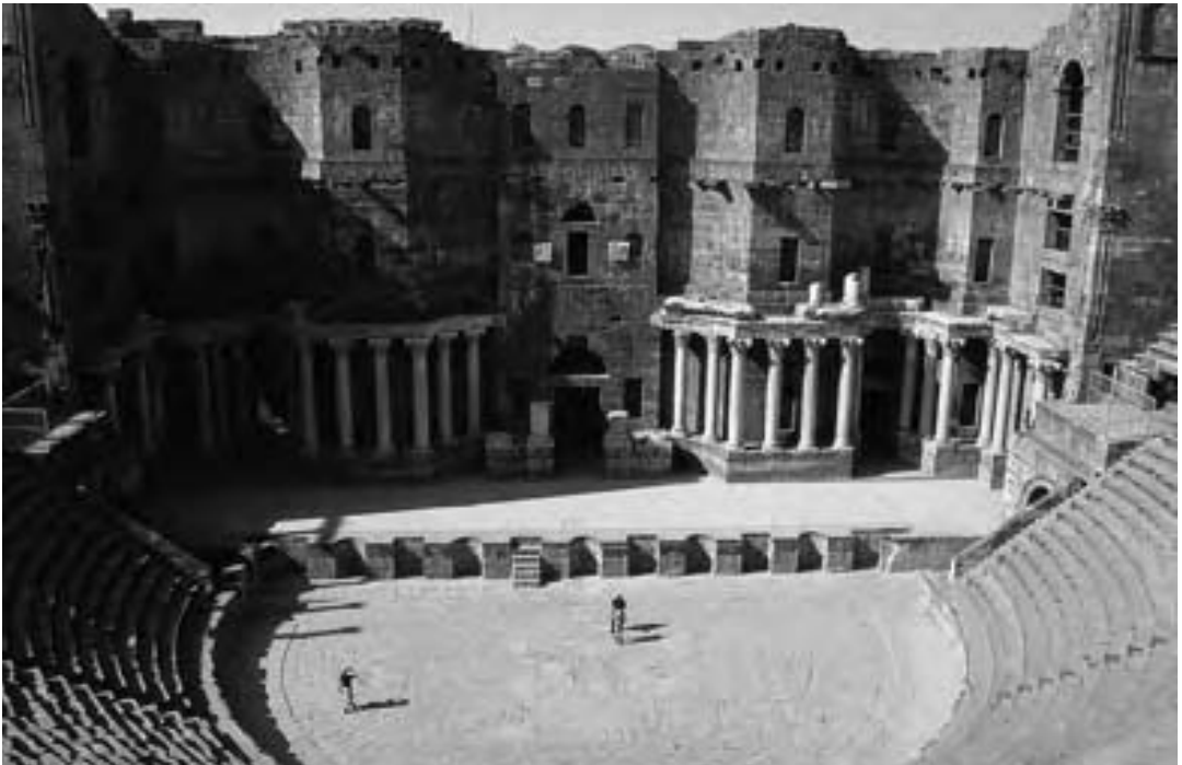
Fig. 24.7 Roman theatre at Bostra, Syria. Local black stone with white marble decoration to the stage building (largely restored). Well preserved because it was incorporated into a medieval castle (Photo: © RAT).
