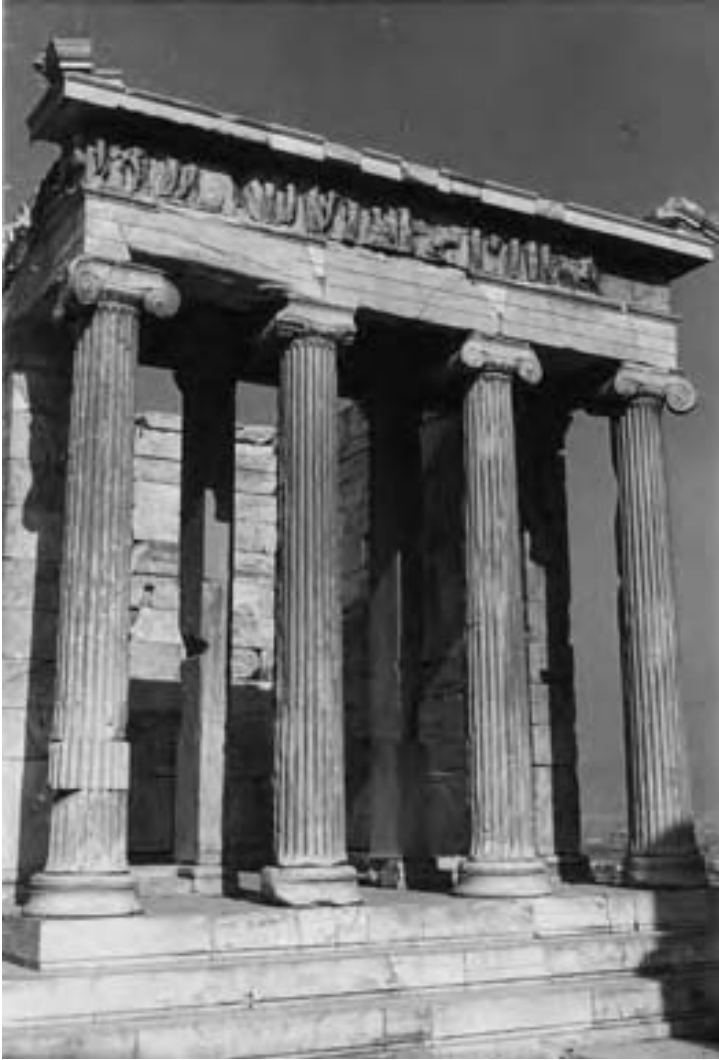
Fig. 24.2 The Greek Ionic order: temple of Nike at the entrance to the Athenian Acropolis, as restored, before the present dismantling (photo: © RAT).
