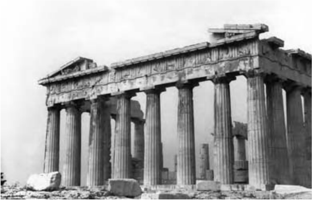
Fig. 24.1 The Greek Doric order: the Parthenon, Athens, before the recent conservation work. Note the curved profile (entasis) of the columns (photo: © RAT).
