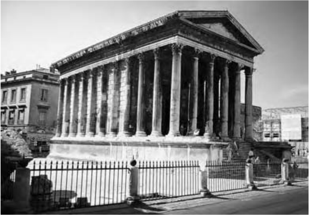
Fig. 24.4 The Maison Carrée, Nîmes. Typical Roman Corinthian podium temple, essentially of metropolitan Roman design, but built in local hard limestone rather than white marble (photo: © RAT).
