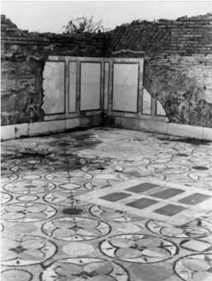
Fig. 24.8 House of Amor and Psyche, Ostia. Marble veneer on brick- and stone-faced concrete walls, opus sectile floor (photo: © G. Lloyd Morgan).
