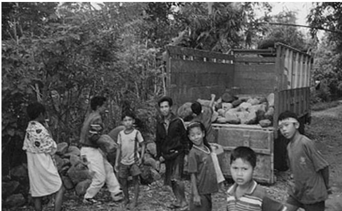
Figure 9.4 Boys collecting stones for construction.
