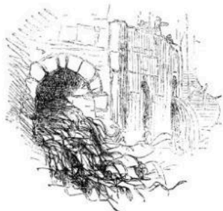
This is the sewer, from cesspool and sink, That feeds the fish that float in the ink- -y stream of the Thames with its cento of stink, That supplies the water that JOHN drinks.
