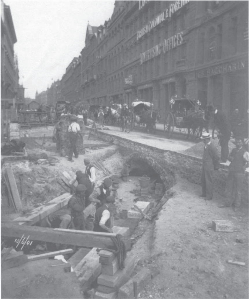
Plate 3.1 The networked city: constructing an underground subway for the Post Office's London Telephone Service, 1901
