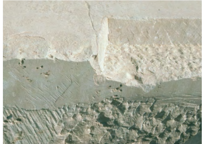
Fig. 6: Persepolis, chiselling of a damaged spot to integrate a work piece; Photo: D. Huff.
