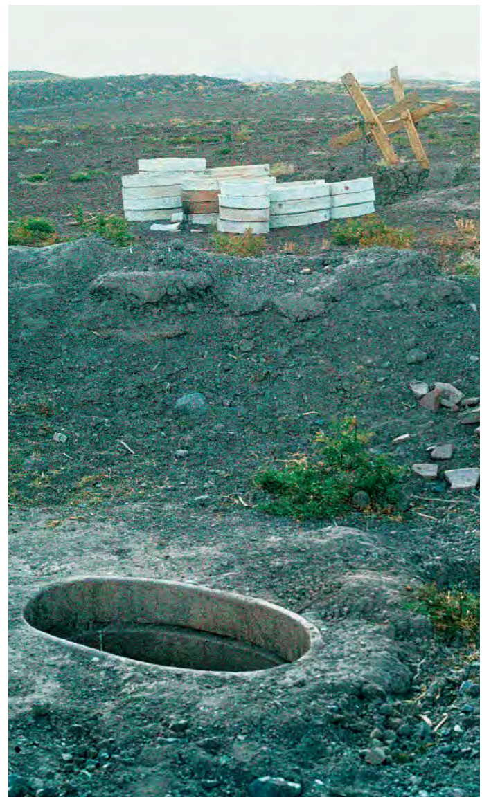
Fig. 4: Near Neiriz, ceramic rings are lying ready for supporting a maybe instable part of the drift or, like in the foreground, for securing a shaft; Photo: G. Weisgerber 1978.
