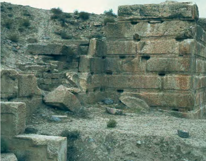
Fig. 1: Pasargadae, Terrace of the palace Tall-i Takht, Greek technique of stonework; Photo: D. Huff.
