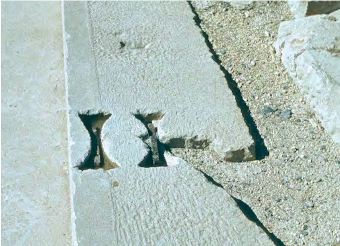
Fig. 5: Persepolis, in lead encapsulated iron staples, located in swallowtail-shaped holes; different techniques of visible and covered stone-surfaces; Photo: D. Huff.
