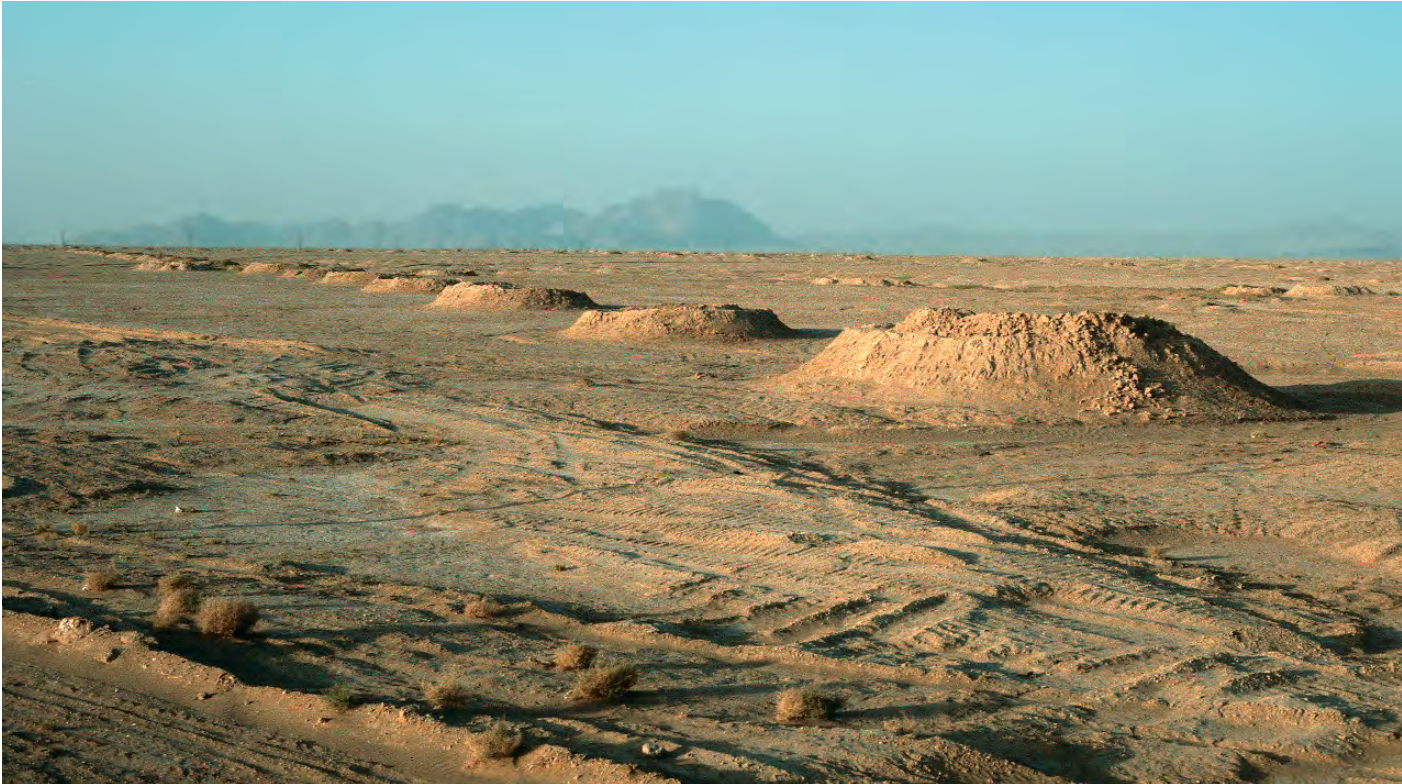
Fig. 2: Seemingly endless, the ring-shaped heaps of various periods of constructing qanat-shafts run from the environments of Yazd to the next settlement; Photo: G. Weisgerber 1978.
