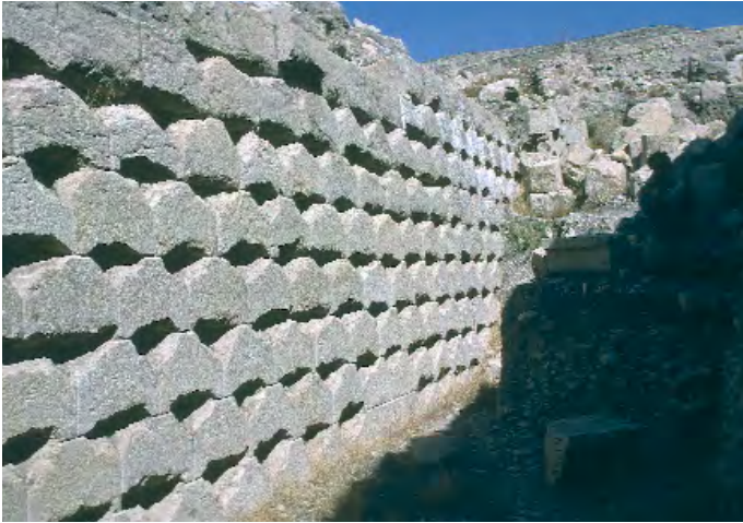
Fig. 10: Bishapur, "Valerian's prison", stonework with ashlar done in Roman technique. The lead was stolen to make bullets; Photo: D. Huff.
