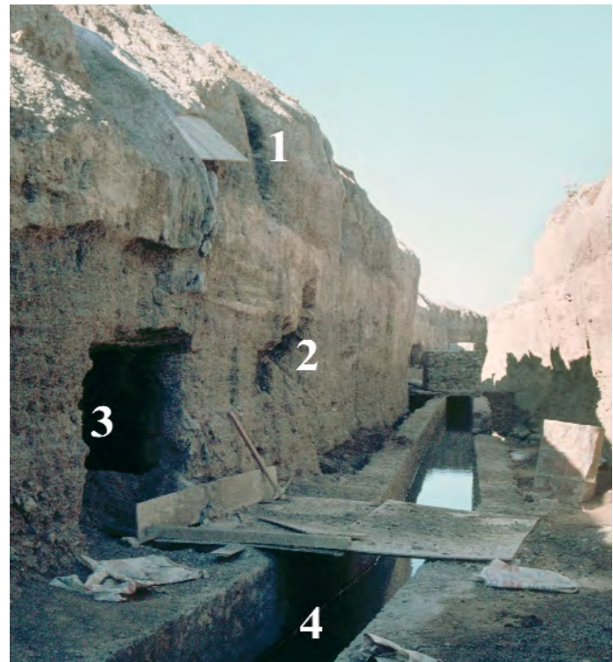
Fig. 9: A recent trench dug by an excavator for securing the transport-section of an Oman qanat near Shareeah revealed several older and long abandoned qanat-drifts which were closer to the surface; Photo: G. Weisgerber 1982.
