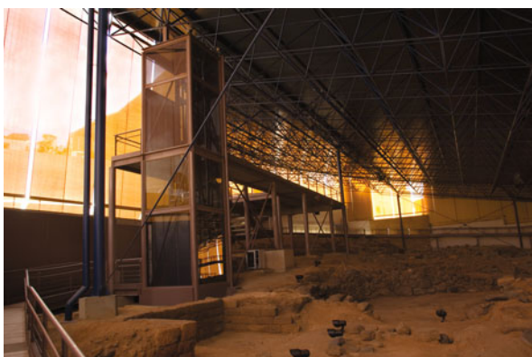
Fig. 4.6 Detail of the first vertical communications node (stairs and lift, essential for access). The site, enclosure, covering, and walkways can also be seen. Photograph: Javier Betancor. ©Cabildo de Gran Canaria
