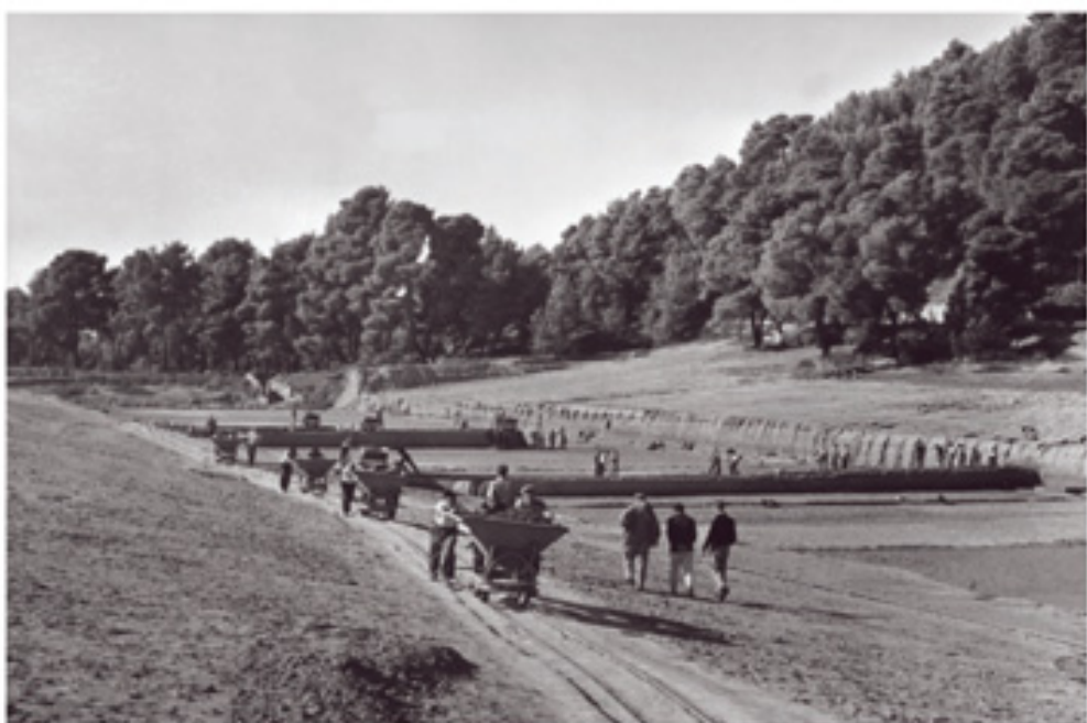
The excavation of the Stadium of Olympia, 1938.
