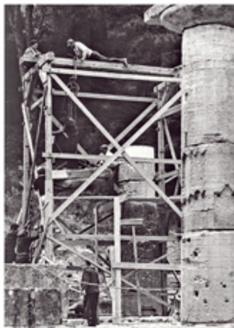
Reconstruction work on the Heronion, 1972.
