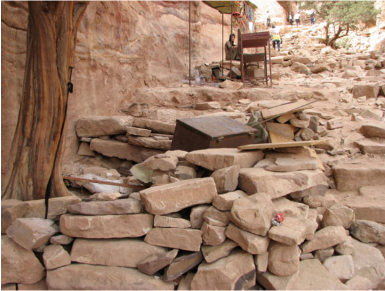
Fig. 1.7 The long, processional stairway that leads to Ad-Dayr has been almost completely destroyed by the feet of donkeys carrying tourists
