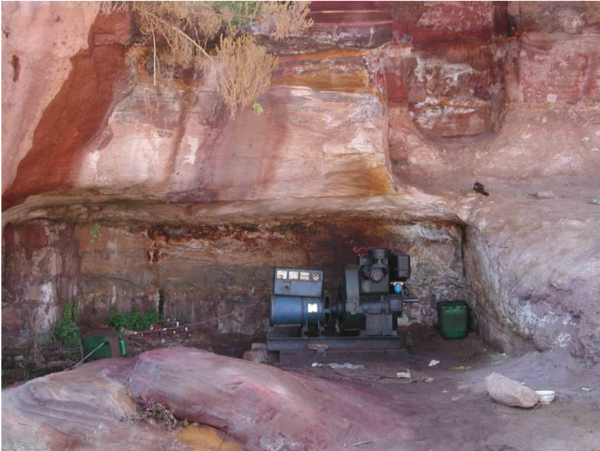
Fig. 2.26 Use of cave as shelter for diesel generator—note oil leakage, 2004 (Courtesy G. Palumbo)
