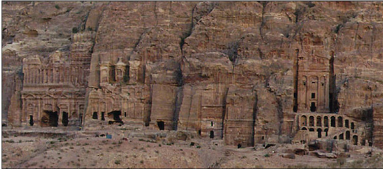
Fig. 5.8 Effect of salt-laden water wicking into sandstone is visible here. This kind of damage occurs from the ground up. Note keyhole shape of tomb entrances
