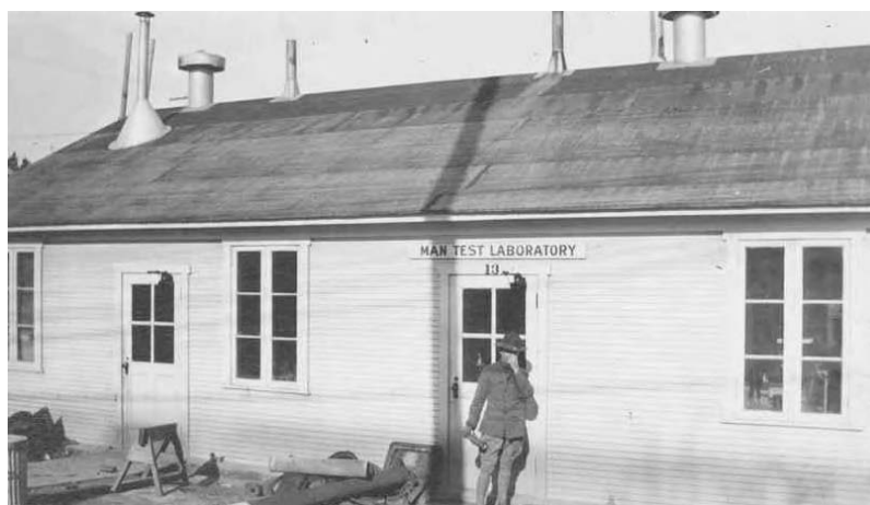
10. Building at AUES where volunteers (presumably including George Temple) were subjected to lewisite skin tests, 1918. Courtesy Addie Ruth Maurer Olson.
