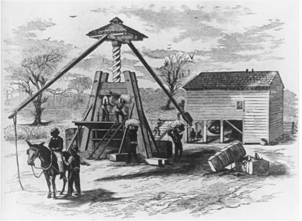
17. Cotton press. Once picked, cotton was packed into bales of approximately 400 pounds. Samples were cut from the bales and distributed to potential buyers. Cotton planters remained liable for damage to their cotton for weeks after it was out of their control. Library of Congress .
