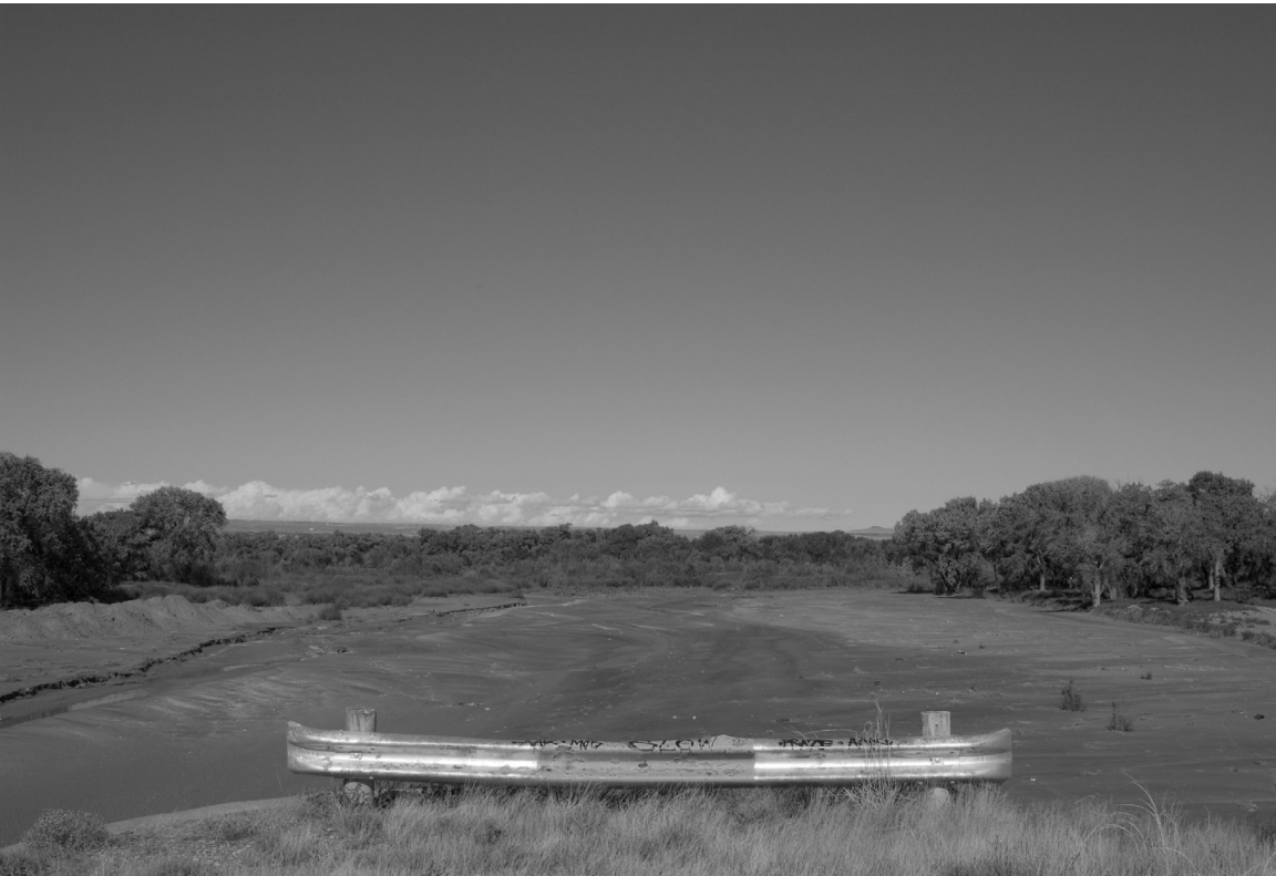
The cement lining of the South Diversion Channel (called the Tijeras Arroyo further up) ends here as it nears the Rio Grande. October 2006.
