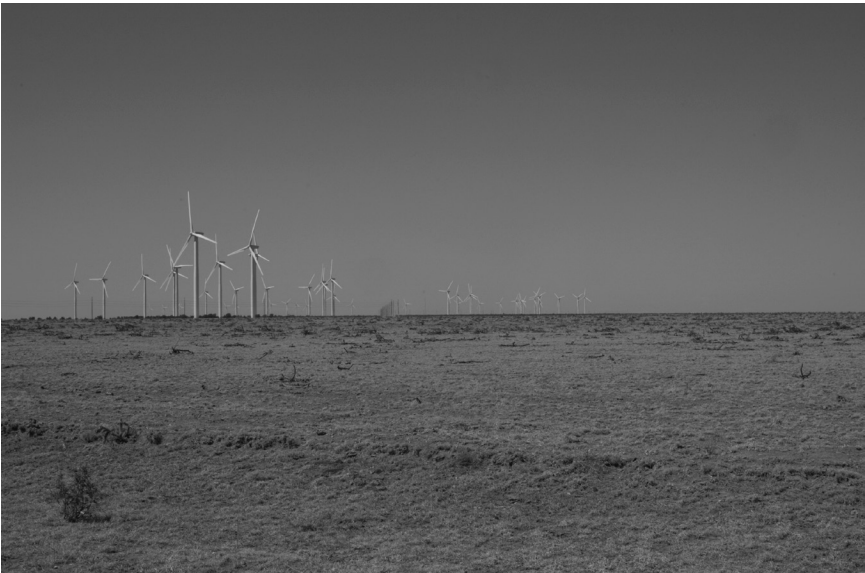
The New Mexico Wind Energy Center near House, in northeastern New Mexico, consists of 136 turbines, each 210 feet tall, with blades 110 feet long. PNM, the state's largest electric company, buys all of the power generated here, which replaces the same amount generated by coal and gas (see page 52). March 2008.
