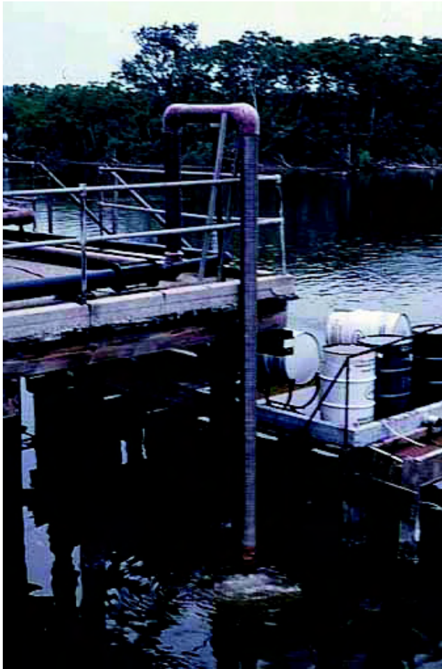
PHOTO 6 Surface water disposal of produced water discharge in estuary of south Louisiana. Water from petroleum-bearing strata (referred to as “produced water”) is recovered when crude oil is pumped to the surface. Although direct disposal is no longer permitted in sensitive coastal habitats in the United States, similar practices continue in other parts of the world. (Photo courtesy of Nancy Rabalais).
