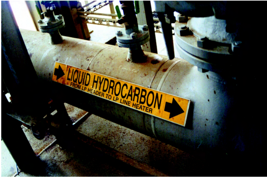
PHOTO 7 Crude oil is heated to maintain low viscosities, thereby making pipeline transport from offshore easier. Low temperatures can also lead to the formation of gas hydrates in pipelines crossing the sea bed. (Photo courtesy of Environmental Research Consulting.)
