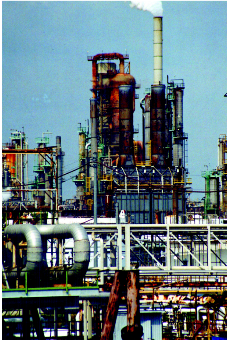
PHOTO 18 Refinery capacity is an important factor in gasoline prices. However, such facilities are also sources of petroleum spills and atmospheric releases of volatile organic compounds that can play a role in local air quality. In the United States most refineries are located near marine transportation terminals along the Gulf of Mexico and the northeastern Atlantic seaboard. (Photo courtesy of Environmental Research Consulting.)
