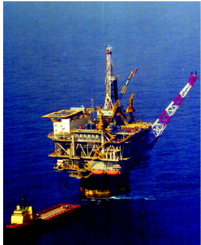
PHOTO 1 The Genesis Spar, located in the Green Canyon 205 Field about 150 miles south of New Orleans, is typical of the new technology allowing oil and gas development in deep waters of the Gulf of Mexico. (The original discovery well was drilled in 1988 in 2600 feet of water.) The Genesis Development Project is a joint venture development between ChevronTexaco Production Company, Exxon Company USA, and PetroFina Delaware, Inc. (Photo courtesy of Environmental Research Consulting.)
