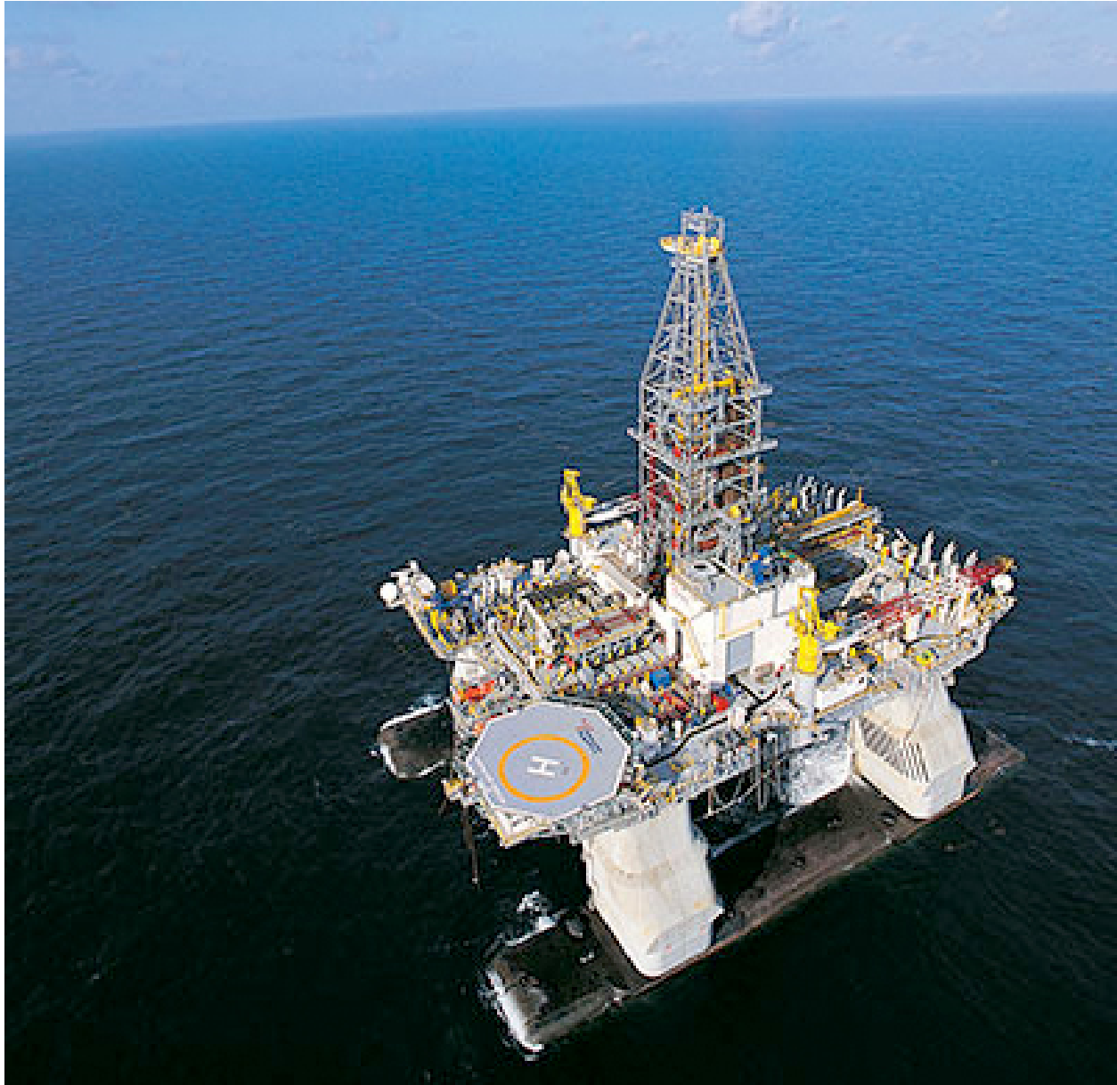
Figure 1.2 – Deepwater Horizon semisubmersible drilling rig. 9
