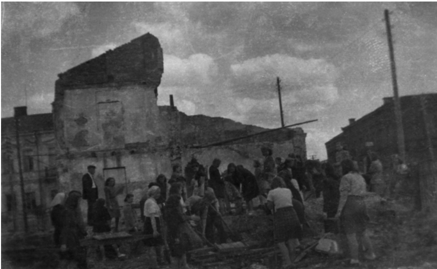
Figure 4 Picking through the war damage
