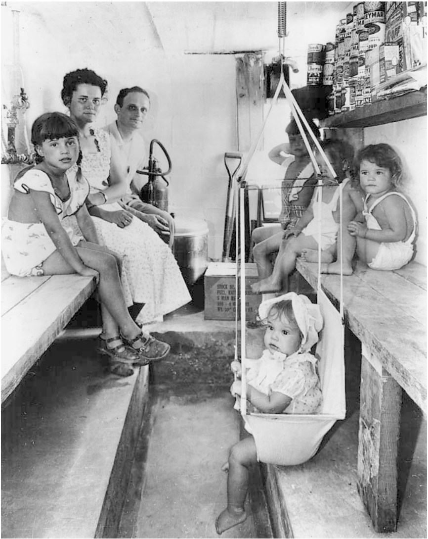
A new portrait of the American family: Harry A. Thomason, his wife, and five children gather in the family's tiny fallout shelter in District Heights, Maryland, in 1955. The family faced the prospect of spending days or weeks in this cramped structure built with reinforced concrete and accessible through the basement. This potential living space for a family of seven was five feet wide, twelve feet long, and just under six feet high. Washington Star photo, National Archives.
