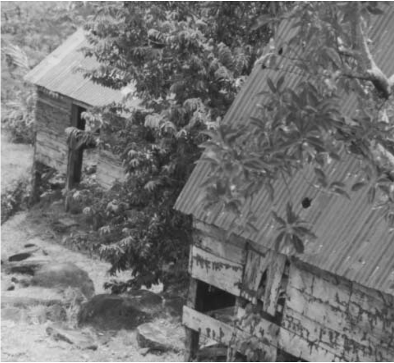
Figure 3: Dilapidated eighteenth-century slave huts on the Habitation La Grivelière
