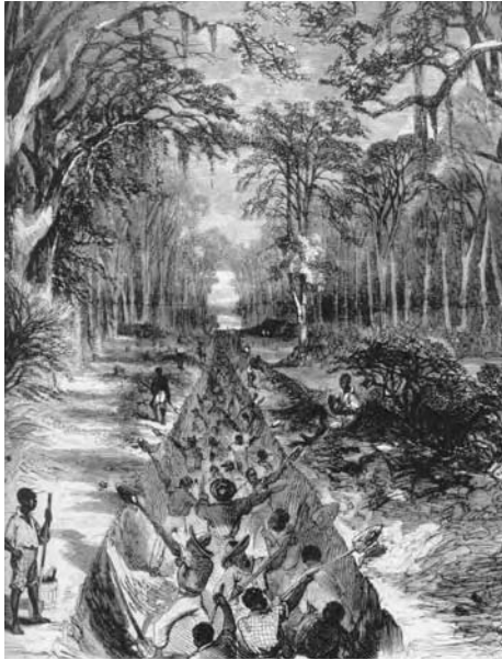
One of the canals General Ulysses S. Grant ordered dug as a means of avoiding the Confederate guns defending the river approach to Vicksburg. From Harper's Pictorial History of the Civil War, 1866
