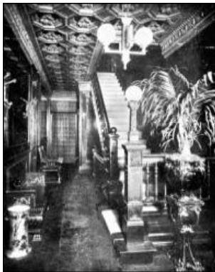
Hallway to the entrance of 2133, the Everleigh Club.
