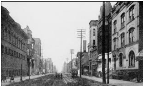
South Dearborn Street. (The Everleigh Club is at near right.)
