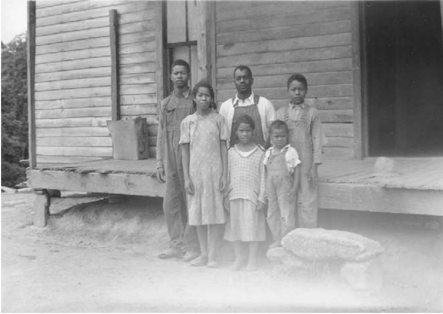
The Mayberry family, North Carolina sharecroppers, had little to their name in 1933. Here they pose for the Resettlement Administration photographer in front of their home, a rundown house with cracks in the walls and a stone for the front steps. Mayberry family, Iredell Co., N.C., 1933. Courtesy of the Franklin D. Roosevelt Library Digital Archives.
