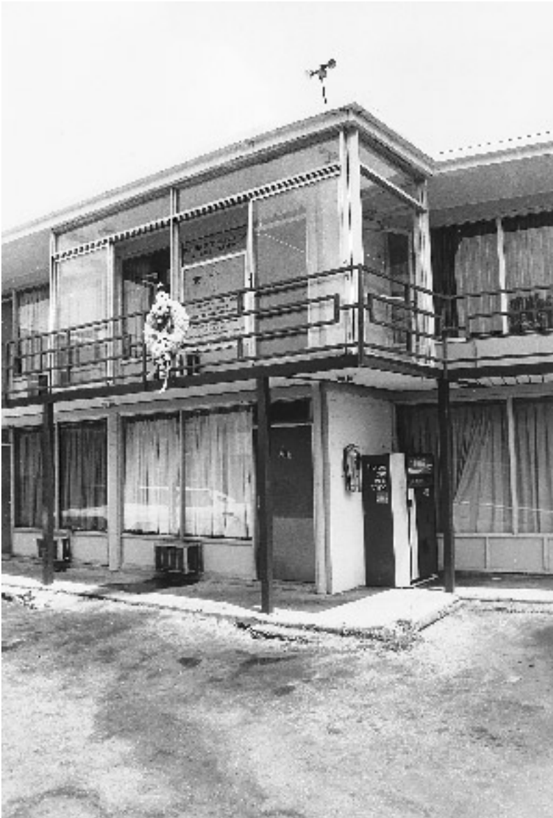
Figure 1-7. The Lorraine Motel in Memphis, Tennessee, looking up toward the place where Martin Luther King Jr. was assassinated on 4 April 1968. The memorial tablet positioned on the wall next to the room Dr. King occupied was erected by the motel's owner.
