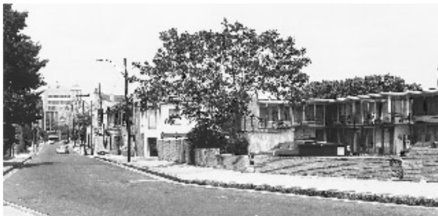
Figure 2-19. The Lorraine Motel in Memphis, Tennessee, in 1986, when planning and fundraising were underway for the National Civil Rights Museum. Walter Bailey, the motel's owner, can be credited with spurring on the effort. The shrine he constructed on the upper balcony helped to elicit subsequent city, county, state, and national support for the memorial. Rather than compete with the King Memorial in Atlanta, the foundation that guided the transformation decided to use the Lorraine to pay tribute to the entire civil rights movement.
