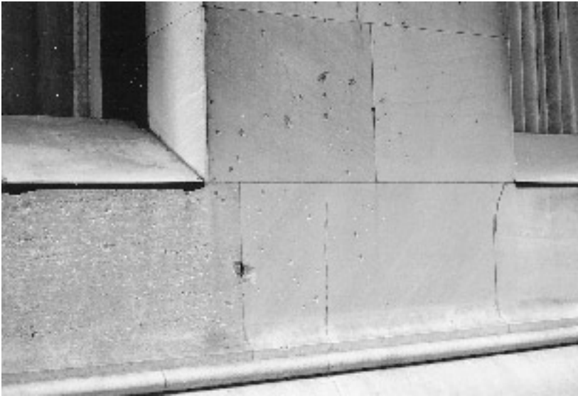
Figure 5-8. Shrapnel scars on a building on Wall Street in New York City caused by the terrorist bombing of 16 September 1920. No one ever confessed to the bombing or was charged with it, and the area damaged by the blast was rectified, as if the explosion had been an accident.
