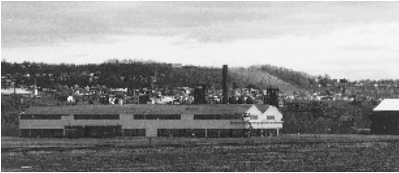
Figure 9-5. The remains of the steel mills of Homestead, Pennsylvania, once one of the nation's largest steel plants and the site of the famous strike of 1892. Plans to commemorate the site are now in debate, but little is left to conserve.
