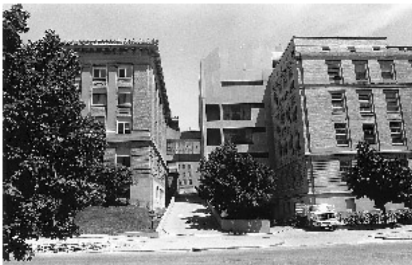
Figure 9-11. The area at the epicenter of the massive bomb that destroyed the Army Mathematics Research Center at the University of Wisconsin in Madison in August 1970. The center was then headquartered in Sterling Hall, the building on the left. The bomb was a protest against university involvement in military research during the Vietnam War and killed one physics researcher. Sanctification or memorialization of the site was never considered. Instead the site was rectified.
