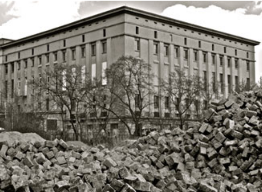
FIGURE 3.6 The iconic architecture of the club Berghain / Panorama Bar that houses the office of its label Ostgut Ton and now also Säule – the club's third dancefloor geared towards more experimental party formats and music gigs. The building is a former power plant located in the district of Friedrichshain, yet close to the border with Kreuzberg, hence the club's name, which combines parts of both district names. Photo by D. Bartmański.
