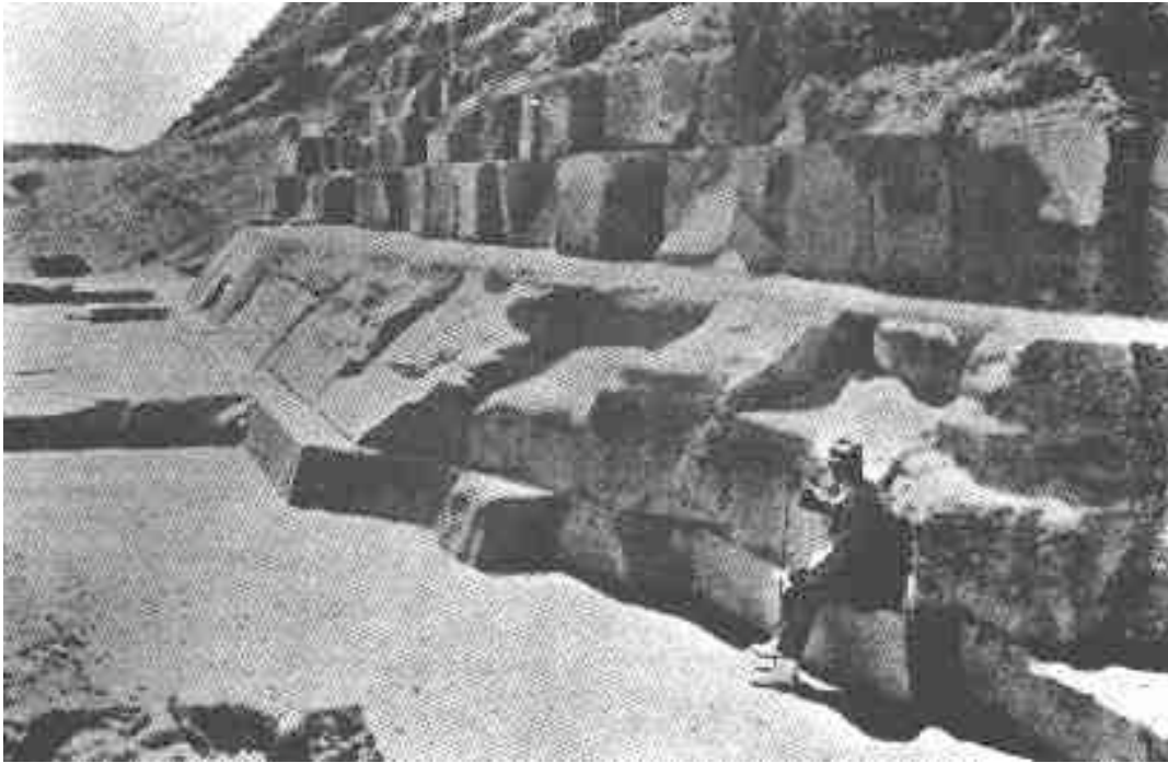
Figure 3.7 – Casing stones that still exist along the base perimeter of the Great Pyramid.
