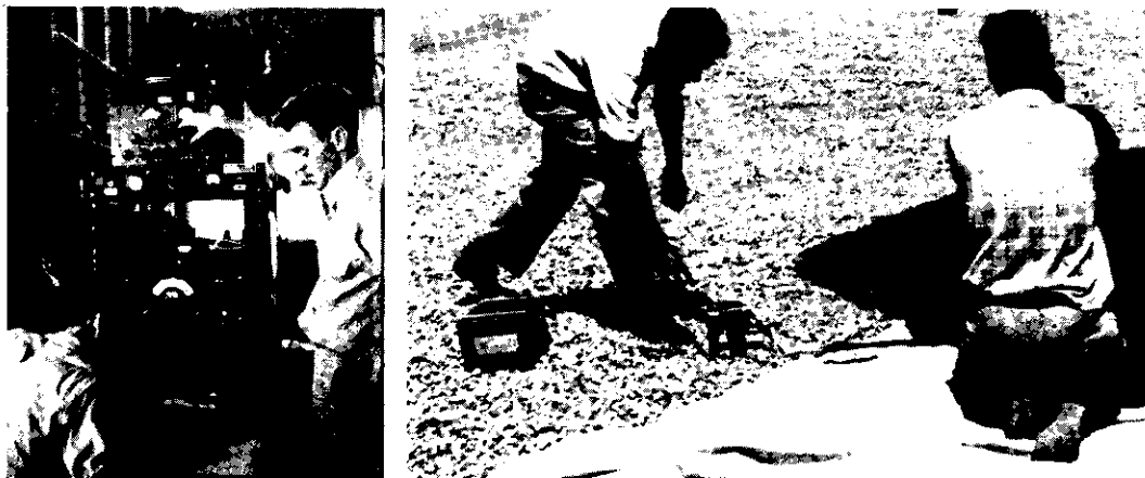
C.B. Moore, New York University Constant Level Balloon Project Engineer ( left and standing ), adjusts an AN/FMQ-1 radiosonde receiver/recorder. The absence of this equipment on the first NYU field trip in June 1947 (it was left behind in New York due to space limitations of the B-17 aircraft) prompted Moore to attach additional ML-307C/AP corner reflectors to MOGUL flights. The addition of the oddly constructed reflectors, intended to enhance radar returns, contributed to the confusion when Mogul Flight No. 4 returned to earth and was mistaken for a part of a flying saucer. Moore ( right and reaching down ) prepares experimental Project MOGUL microphones for launch (Holloman AFB, Alamogordo, NM, July 1948).
