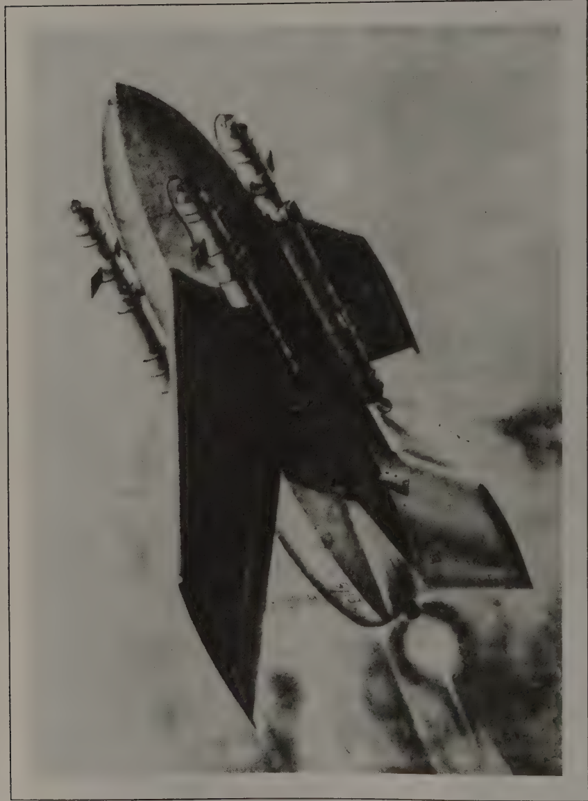
Enzian 4 in flight. This was an exceptionally powerful rocket intended to reach supersonic speed, a ceiling of 52,000 feet, and distant targets under radio control. It is but one of many missiles produced by the German secret weapons program (courtesy of "German Secret Weapons of World War II" by I. V. Hogg, 1970).
