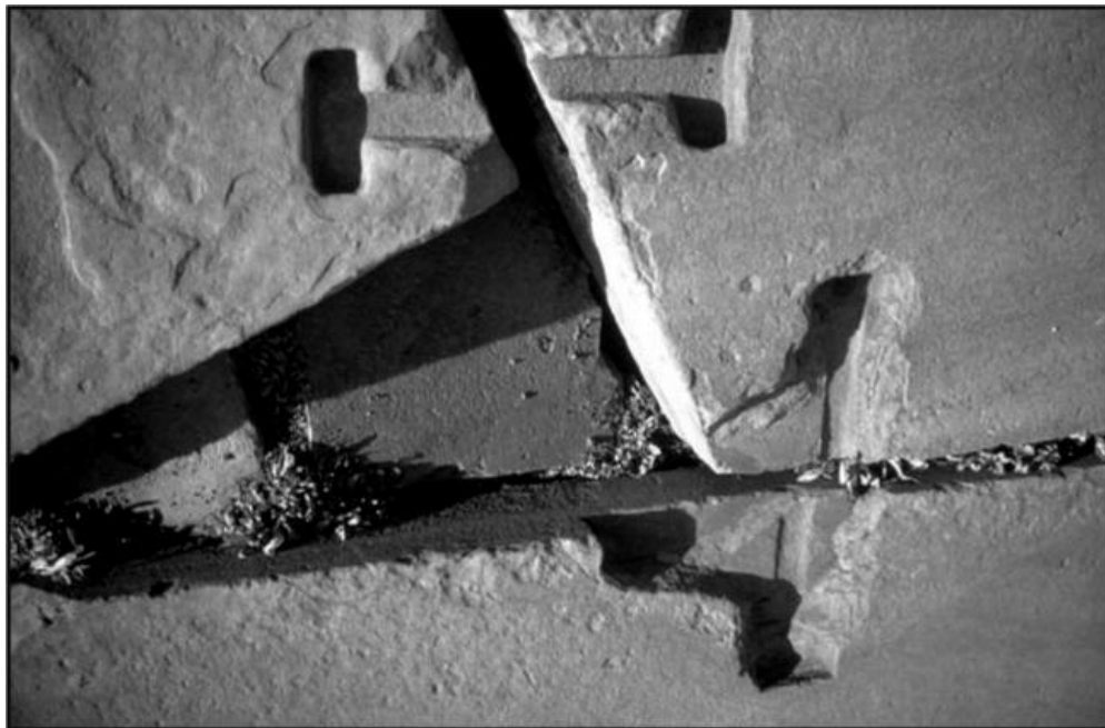
1.20. The slabs were originally held together with fastenings. Image courtesy of Tatjana Ingold, Solothurn, Switzerland.
