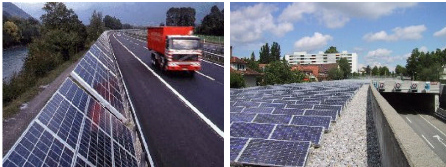
Figure 6-3: PV integrated in noise absorption (left) and as roofing of a highway (right)
