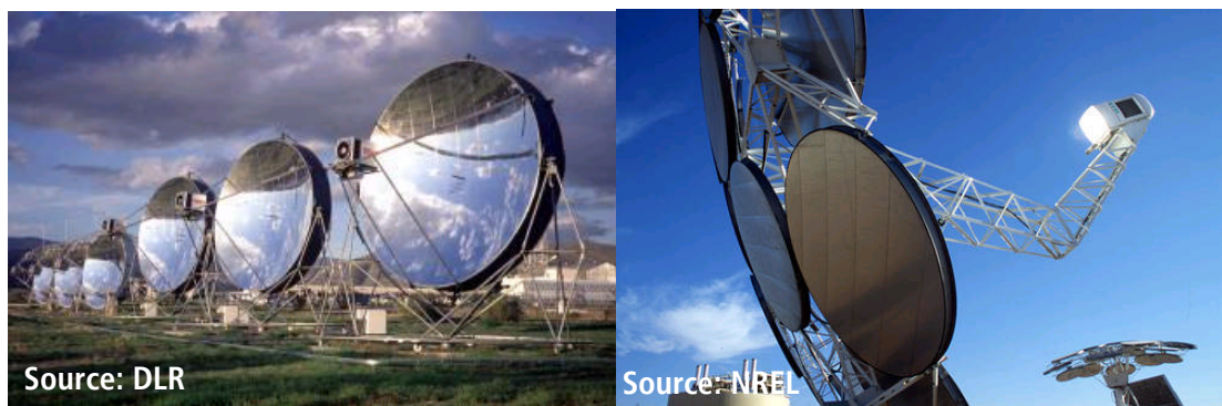
Figure 2-37: Solar Dish: left: parabolic dish installations, source: [DLR SOT]; right: solar dish plant in Arizona [NREL 2003].
