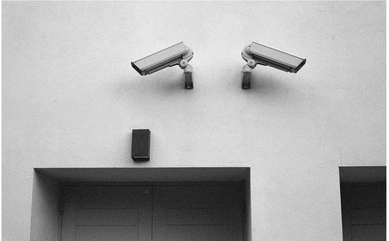
Surveillance cameras help police identify and track down criminals. (Steve McDonough/CORBIS)
