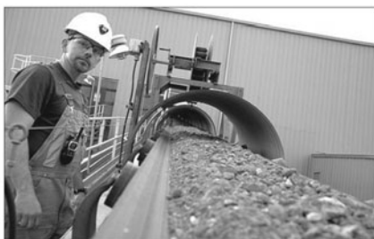
Work at Washington state's Buckhorn mine, one of three growth projects that has helped Kinross Gold.
