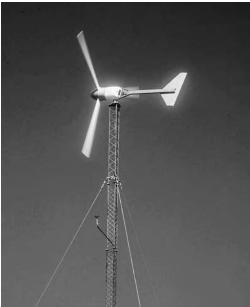
The 10 kW Bergey wind turbine at Inn Serendipity, placed on a 120-foot (37 m) guyed lattice tower.
