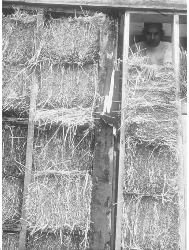
Straw bales stacked as organic infill for greenhouse walls at Inn Serendipity.
