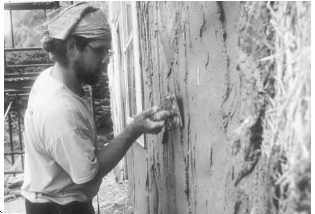
Scratch coat application over straw bales.
